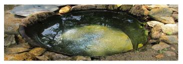
The Kuruma tribe (a native tribe of Wayanad) uses a special type of well, called the panum keni, to store water. Wooden cylinders are made by soaking the stems of toddy palms in water for a long time so that the core rots away until only the hard outer layer remains. These cylinders, four feet in diameter as well as depth, are then immersed in groundwater springs located in fields and forests. This is the secret behind how these wells have abundant water even in the hottest summer months.
